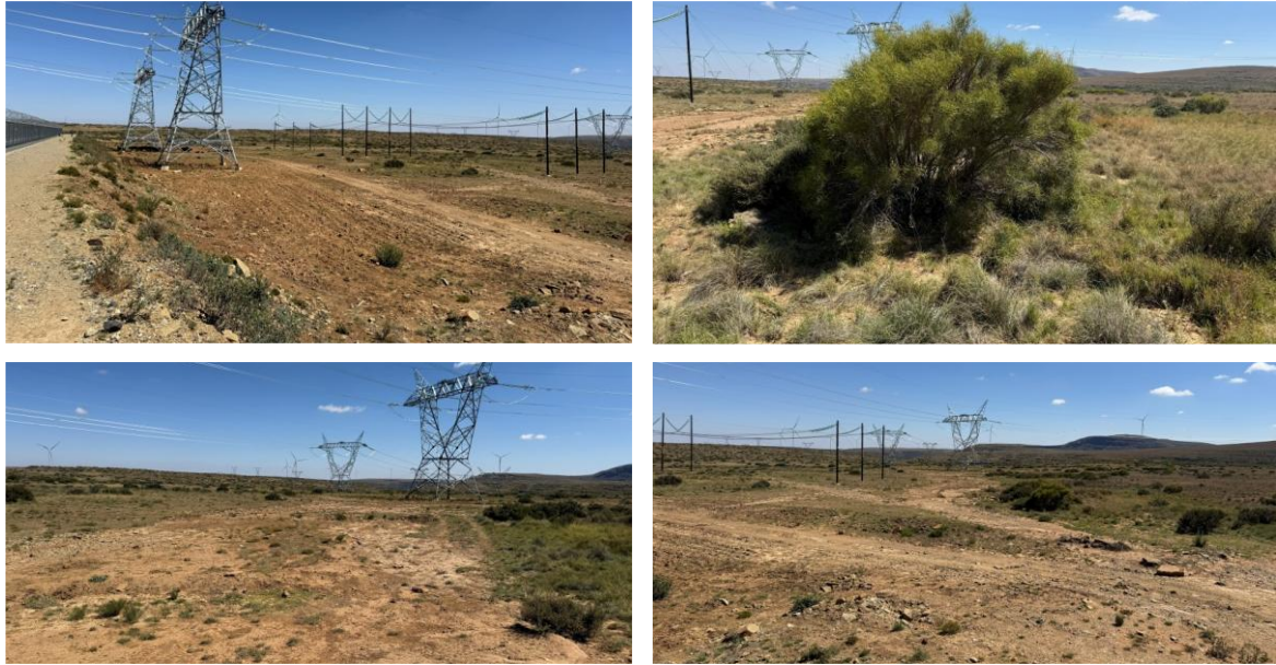
Figure 6-2: Current Condition of the Preferred SynCon Installation Site.
