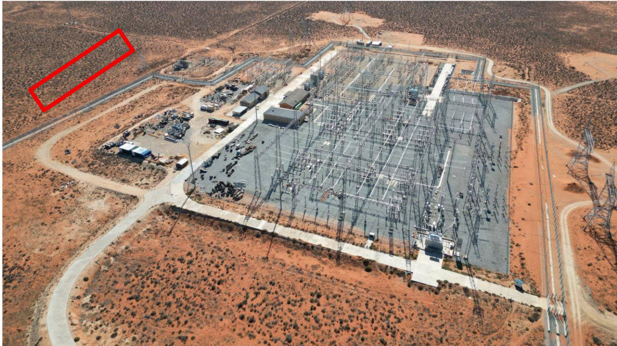
Figure 6-4: Overview of the potential laydown area.
