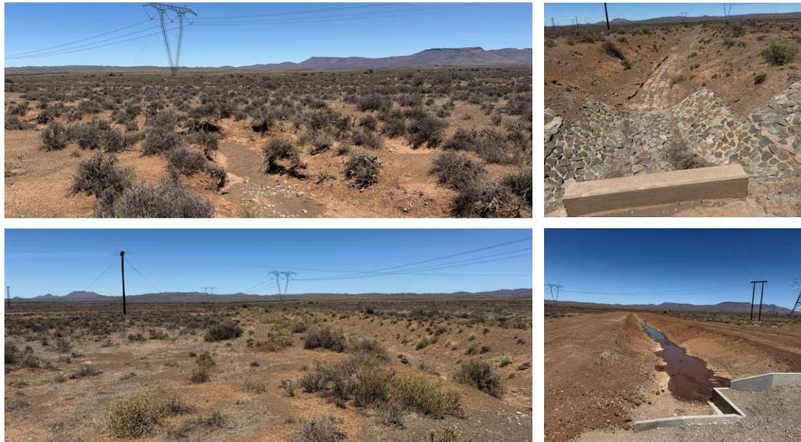
Figure 6-2: Drainage lines and associated stormwater management infrastructure.
