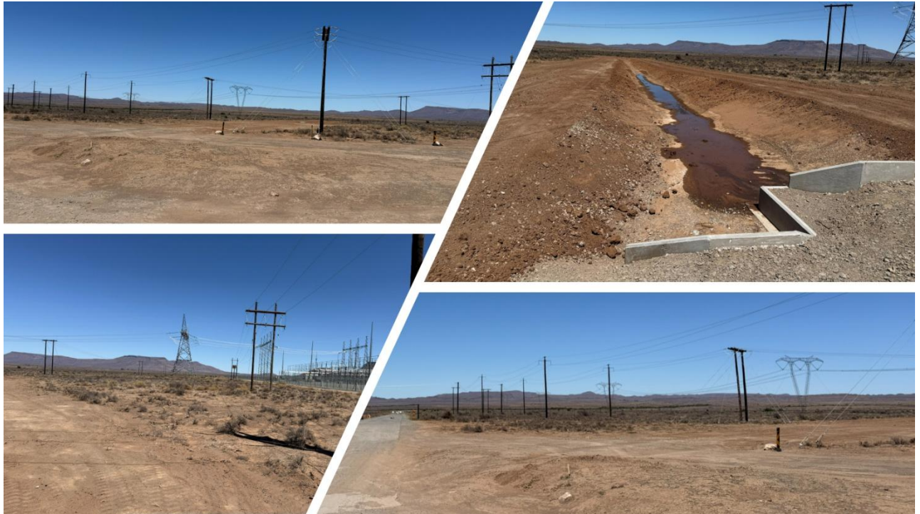
Figure 6-2: Overview of the preferred synchronous condenser location, showing evidence of ongoing anthropogenic disturbance.
