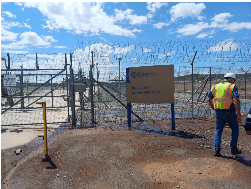
Figure 4: Existing Gamma Substation
