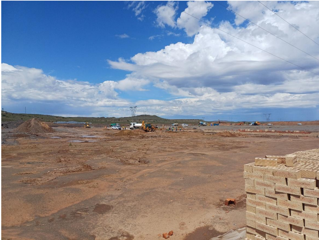
Figure 5: Construction Activities near the site
